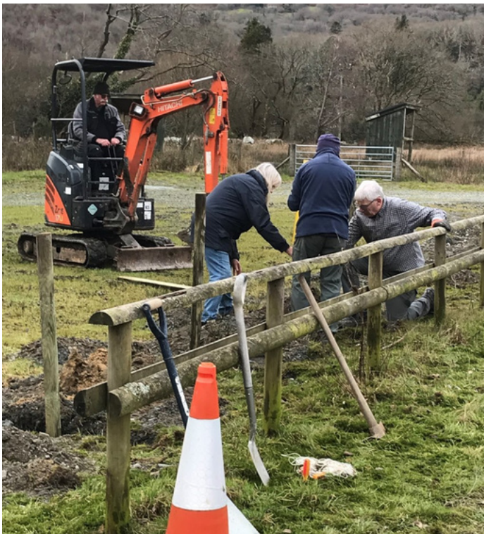
WORK UNDER WAY ON THE CAR PARK
